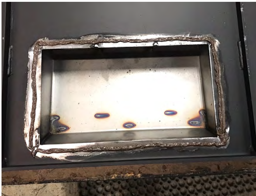
Cement bead around catalyst opening
